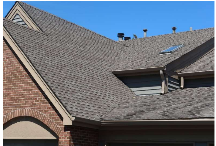
Asphalt shingle overview
