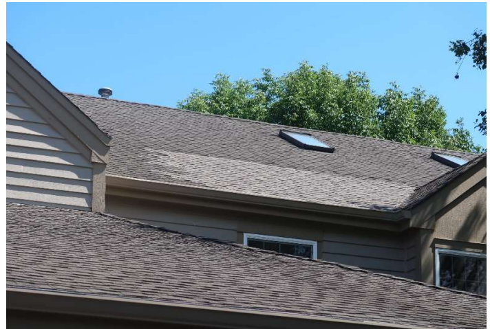
Evidence of roof repair
