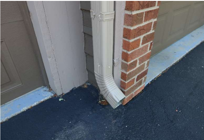
Downspout termination at grade
