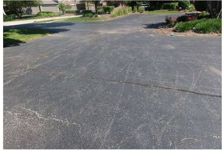
Asphalt pavement overview
