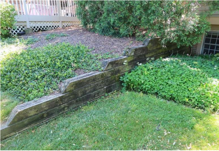
Timber retaining wall overview
