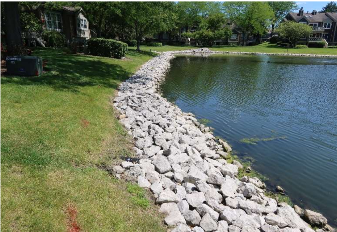
Typical rip rap in good condition
