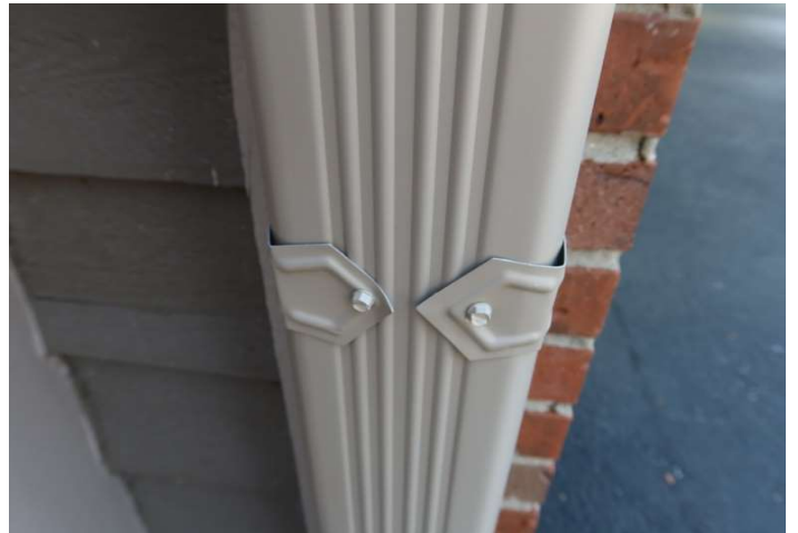
Downspout finish in good condition
