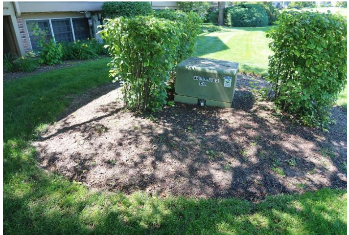
Lack of mulch at landscaped area
