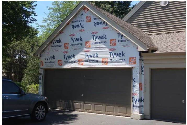
Building façade renovation
