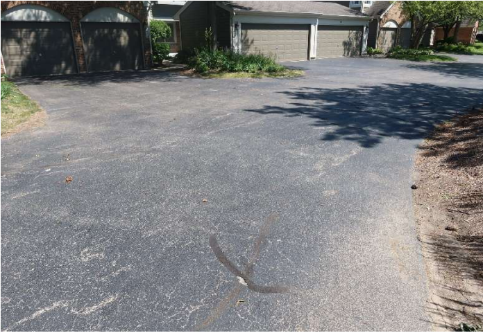
Asphalt pavement overview
