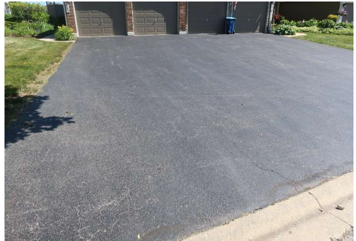
Asphalt pavement overview
