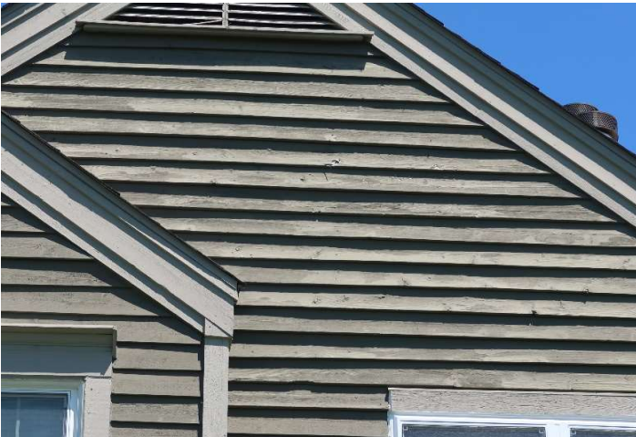
Typical wood siding in fair condition
