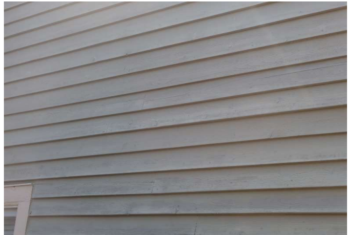
Typical paint finishes at wood siding
