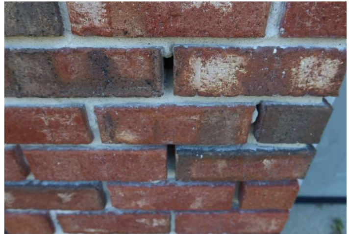
Eroded mortar
