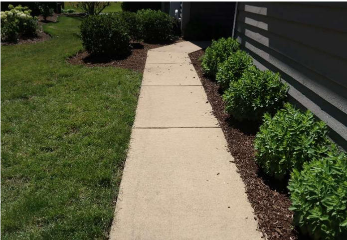
Concrete sidewalk overview
