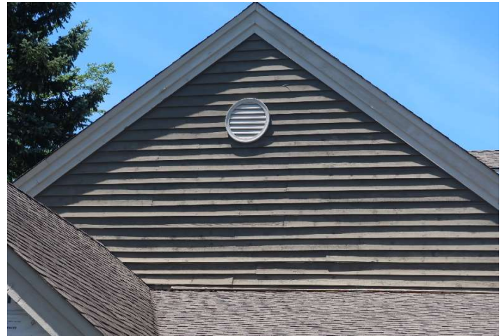
Wood soffit and fascia overview
