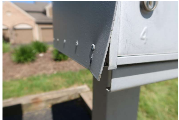
Damage at mailbox station
