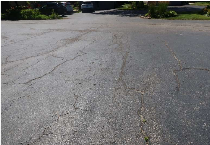
Asphalt pavement overview
