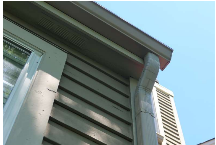
Gutter and downspout overview
