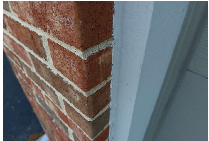
Typical sealant at garage door surround
