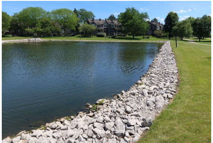
Typical rip rap in good condition
