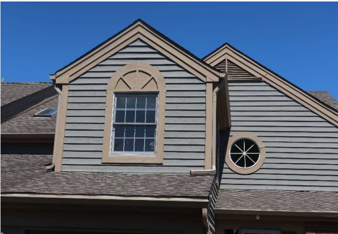
Wood soffit and fascia overview
