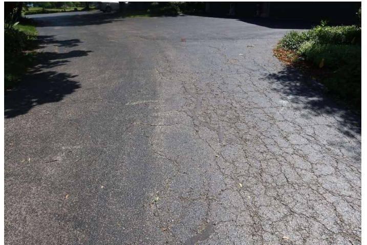
Alligator cracking
