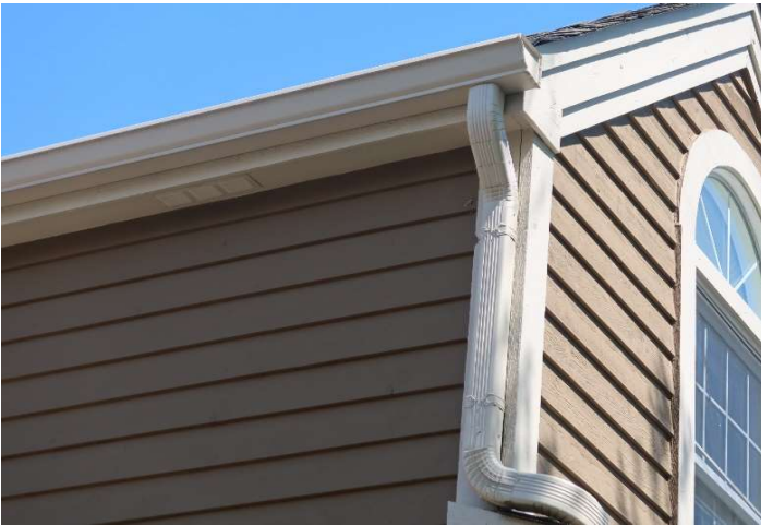
Gutter and downspout overview
