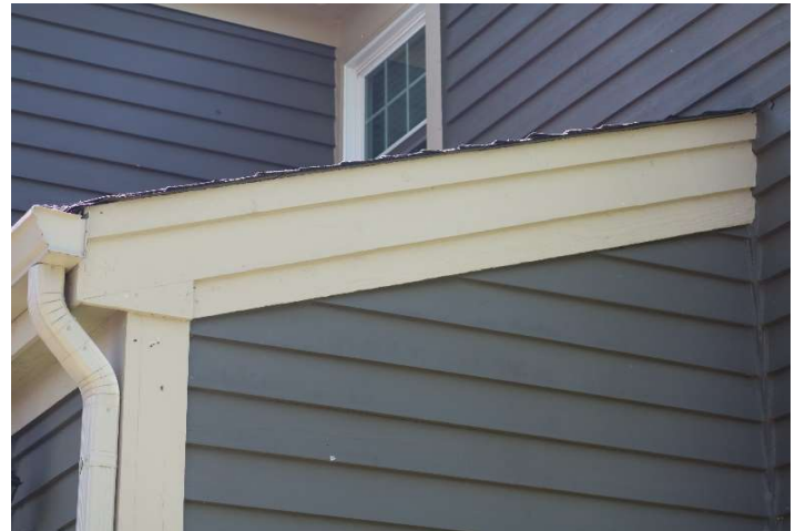
Wood fascia in typical condition
