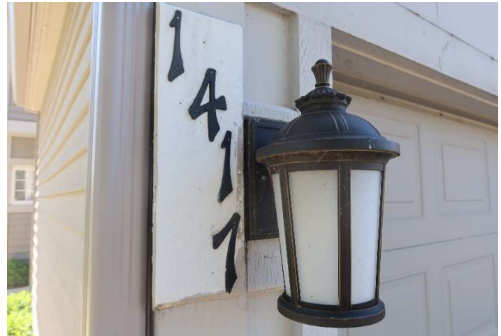
Typical light fixture at garage façade
