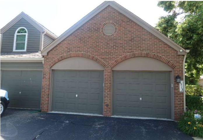
Masonry wall overview
