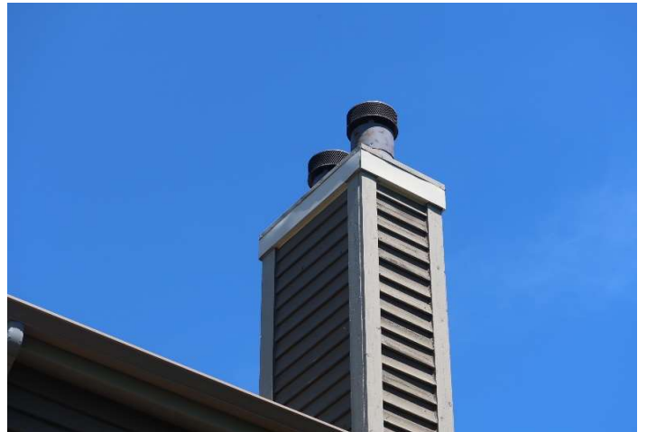
Chimney cap in typical condition
