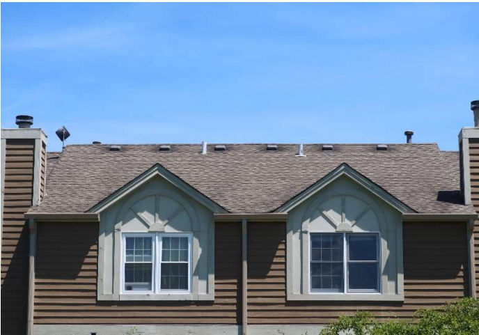
Asphalt shingle overview
