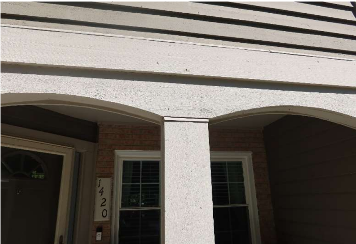
Wood trim at unit entry
