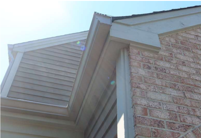
Wood soffit in typical condition
